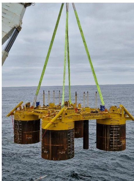
Bestla Subsea Template being lifted from the installation vessel and slowly submerged towards its final position.
